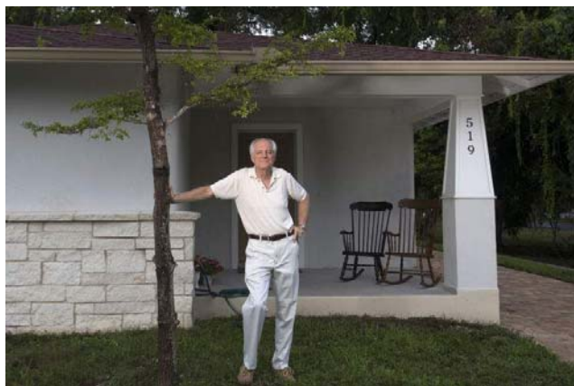
Figure 1: Bob Clayton crafted a 1,640-square-foot house of hempcrete — the hemp plant's woody core and a lime-based binder. Photos by JOHN PENDYGRAFT | Times-Hempcrete house in Florida
